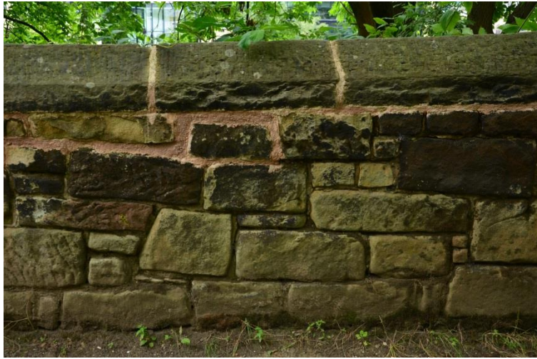
Ashlar Wall on Hume Walk
