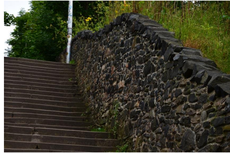
Rubble Wall on Steps from Hume Walk
